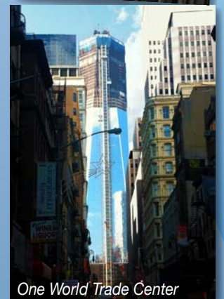
Gehry with Woolworth Building in mirror
